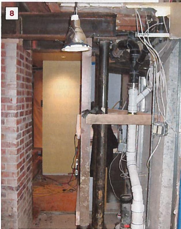
The channel created for the beam was about an inch too high (6), but the space would be filled later with stone shims and non-shrink grout. For now, it gave us the needed clearance to make the installation easier. We hoisted the first beam with our Genie lifts, positioned it (7), and bolted it to the post caps at each end while our temporary supports were still in place (8).
